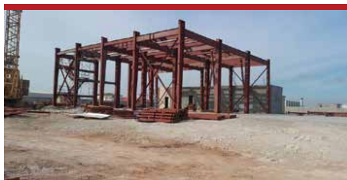
Fish Food Processing Factory - Algeria
