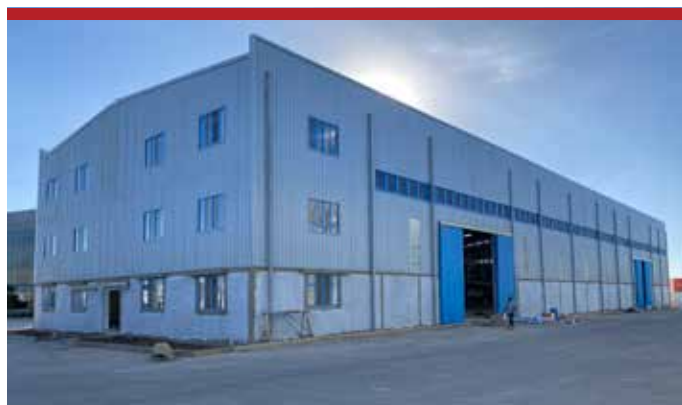
View of building with cladding
