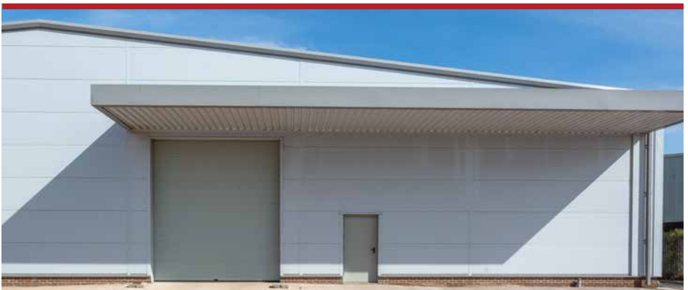
Canopy with soffit panels
