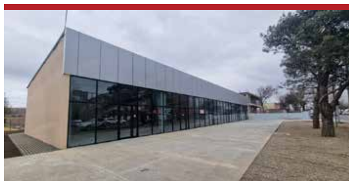
Warehouse and Showroom - Georgia
