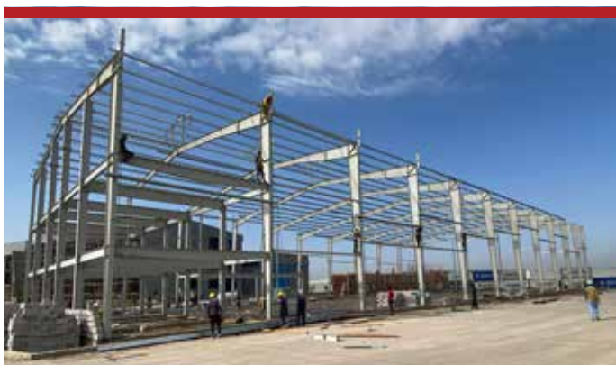
View of building without cladding
