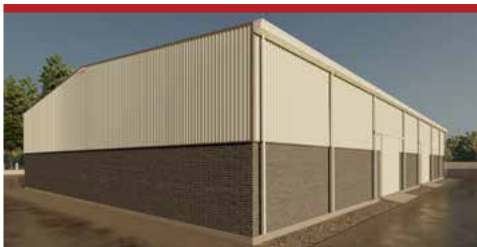
Ceramics Storage Building - Argentina
