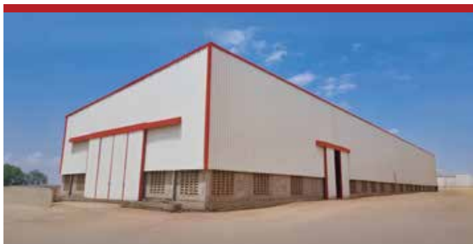
Pipe Factory - Tanzania
