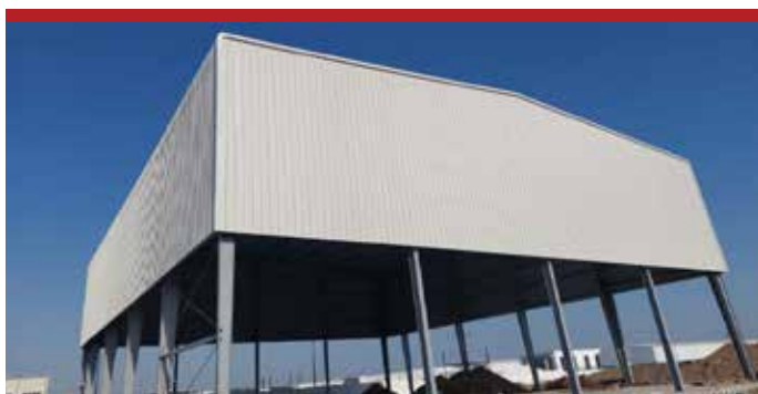
Calcium Carbonate Manufacturing Plant - Oman
