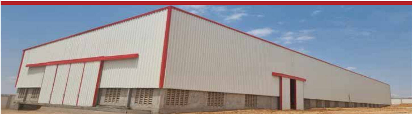
Pipe Factory - East Africa
