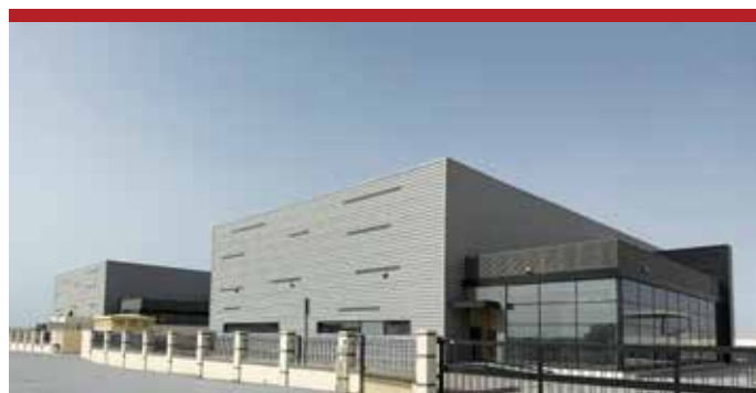
Warehouse and Office Facility - UAE
