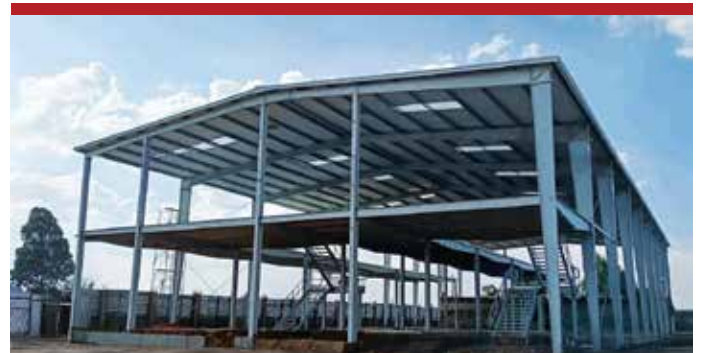
Avocado Processing Facility - Kenya
