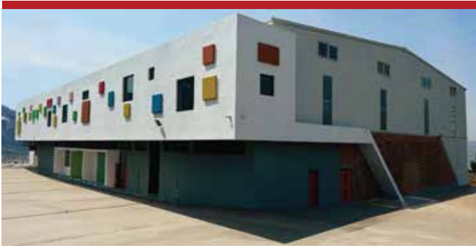
Sports Hall - Rwanda
