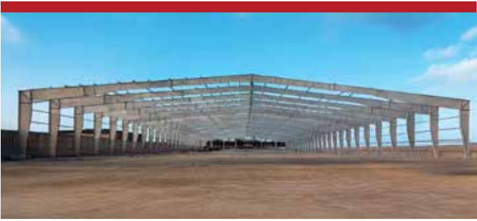
Pre-Engineered Steel Buildings
